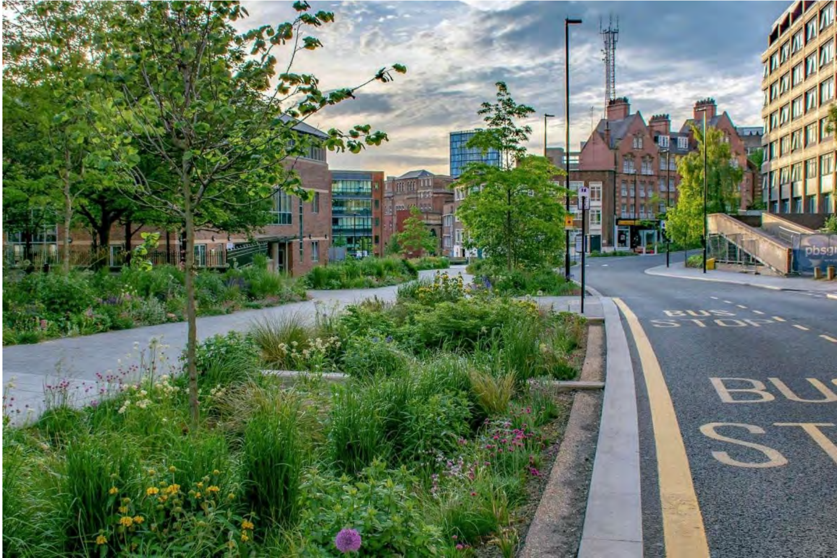
Sheffield, UK: Permeable lane surfaces, planters, rain gardens for stormwater management.
